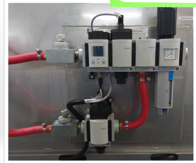
ATMOSPHERE GAS CHAMBER
