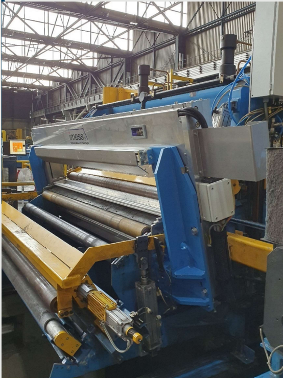
Installation in the roll cage
